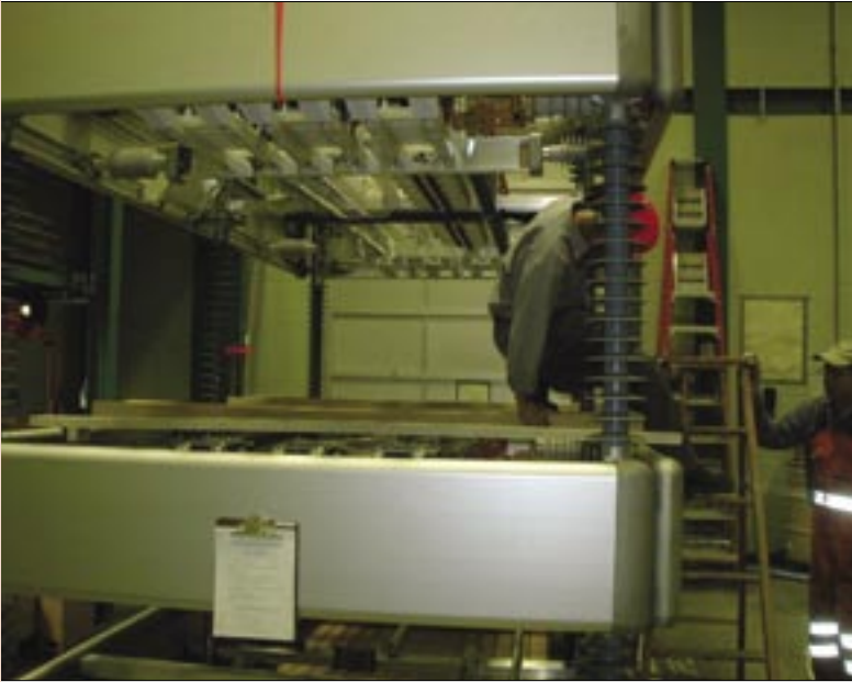
Because of its height, this thyristor exposes workers to the danger of falling more than 2.5 metres. Right: Design details for a fall protection safety net for the thyristor.
