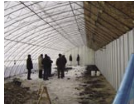
Solar greenhouse at Elie, Manitoba, under construction December 22, 2004. Although the temperature that afternoon was -22^{\circ}\text{C} , with winds gusting to 20 km/h, the temperature inside the greenhouse was a promising -1^{\circ}\text{C} .
