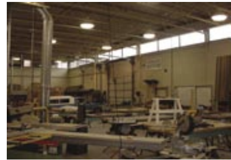
Metal halide lighting now supplies roughly six times as much light in the Carpentry Annex.
