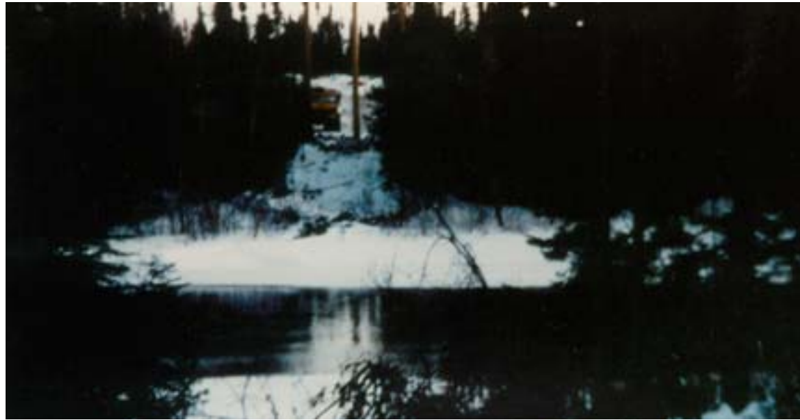
Top: Snow and Ice ramp under construction at a water crossing on Island Lake at St. Theresa Point. This is a standard construction practice to create a working surface that protects sensitive shoreline soils from the heavy equipment needed to install a river crossing. Bottom: Clearing at a river crossing on the North Central Project. The narrow cleared section through the trees is only 8 feet wide — the bare minimum needed to pull the conductor through for stringing on poles. Such a narrow swath grows back within a season to maintain the tree buffer which anchors shoreline soils, protecting against erosion and minimizing visual impact. The standard width of the right-of-way here is 125 feet.
