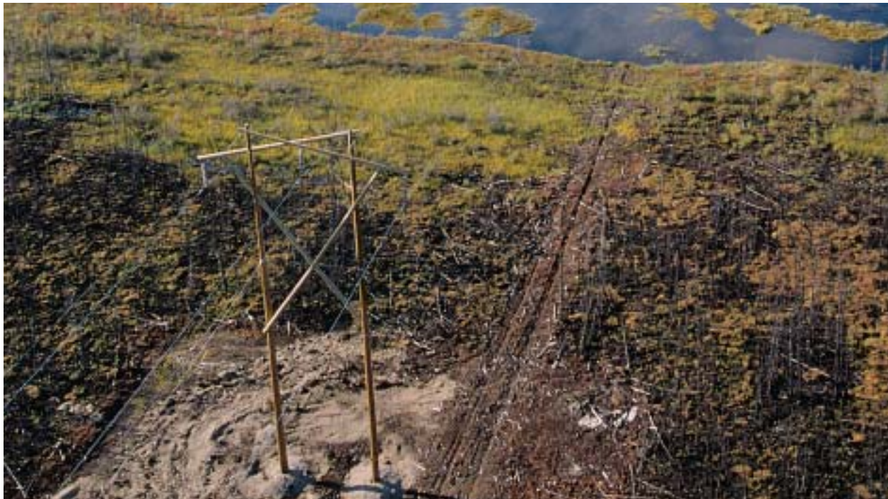
Photo Left: One of the transmission lines that serve communities on the North Central Project.
