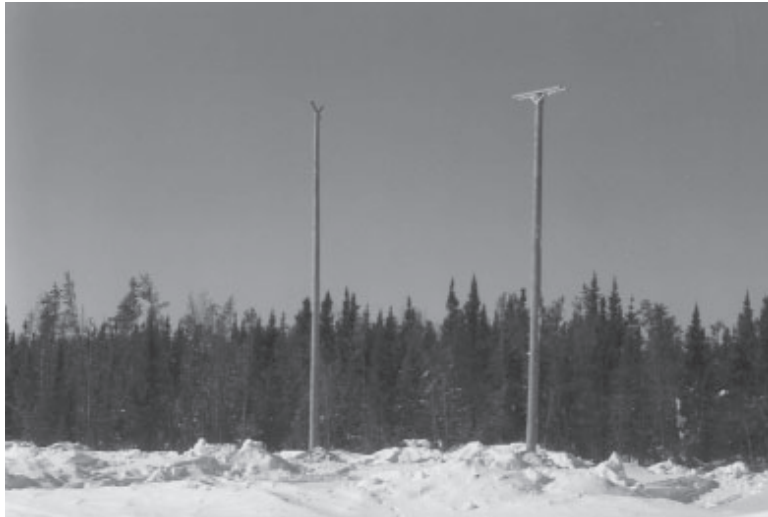
Perching poles and nesting platforms are erected to attract birds away from transmission lines and structures and station poles. They are taller than surrounding structures.
