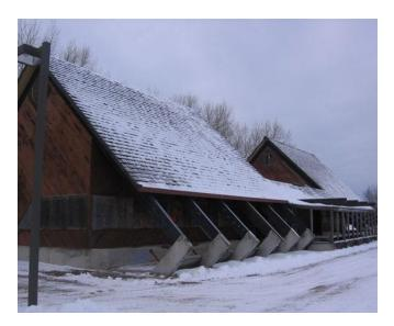
Although heat has been maintained during the winters, inspections have revealed extensive mould growth, mechanical and electrical systems in complete disrepair, deterioration of the building envelope, and evidence of asbestos insulation.
