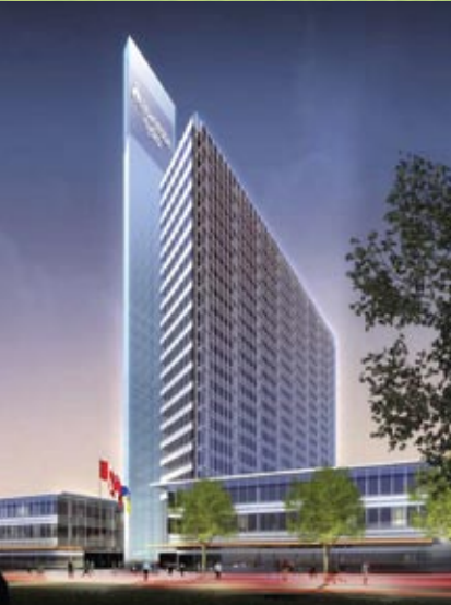
Manitoba Hydro's new energy-efficient head office is under construction in downtown Winnipeg
