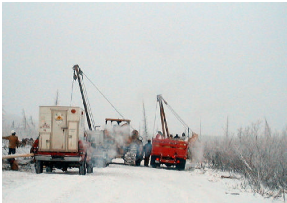
Laying the Ikhil Pipeline to Inuvik
