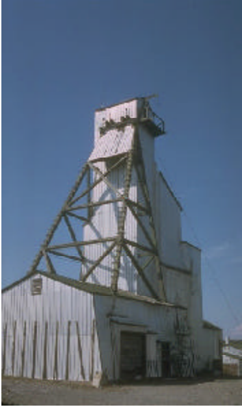
Gold mine headframe
