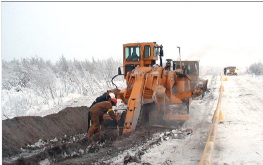
Laying the Ikhil Gas Line to Inuvik
