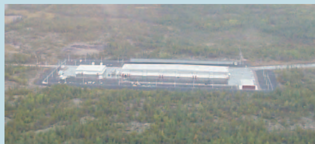
The Department of National Defence (DND) operates the Canadian NORAD Region (CANR) Forward Operating Location (FOL) situated to the southwest of the airport site. The FOL Yellowknife is a personal accommodation barracks and a hangar facility for the CF-18's deployed by the Canadian Air Force.
