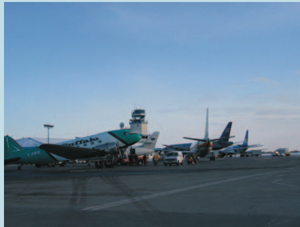
The existing PTB aircraft parking apron is reaching capacity. Reconfiguration and minor expansion of the main apron is underway to meet increased commercial aviation traffic.
