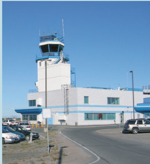
The YZF air traffic control tower provides airport and ground control services to pilots approaching and departing the airport. NAV CANADA's Flight Service Station (FSS) is also located in the PTB, below the air traffic control tower.
