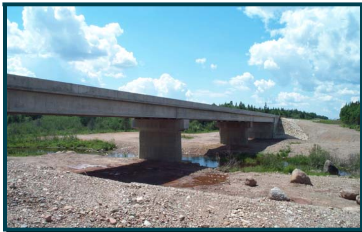
Junction Brook Bridge, Trans Canada Highway, East of Deer Lake
