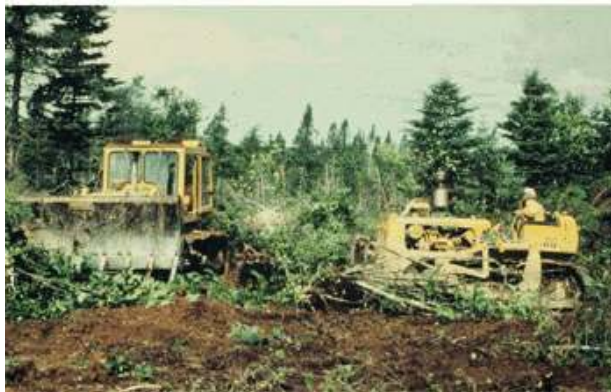
Figure 2. The ‘Walkdown and Pile’ method.
