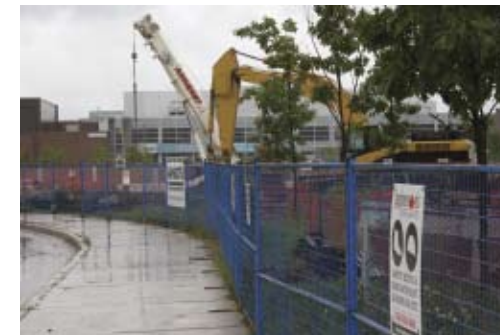
Construction has begun on "The Automotive Centre of Excellence" at VOIT.
