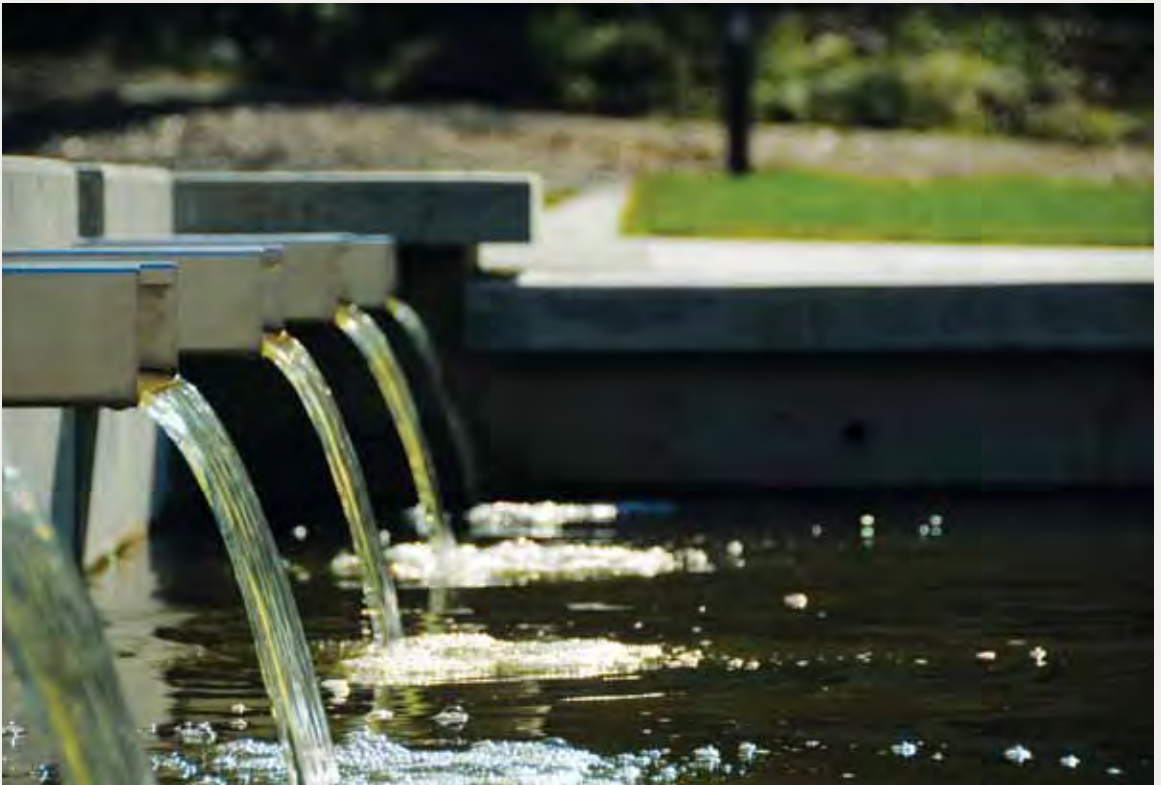
ABOVE: THE NEW WESBROOK PLACE COMMUNITY FEATURES A SERIES OF PONDS AND CHANNELS, ALLOWING DECANTING AND INFILTRATION OF WATER INTO THE AQUIFER FOR STORAGE AND RE-USE AS IRRIGATION—ENSURING THAT RAIN IS TREATED AS A RESOURCE RATHER THAN AS WASTE.
