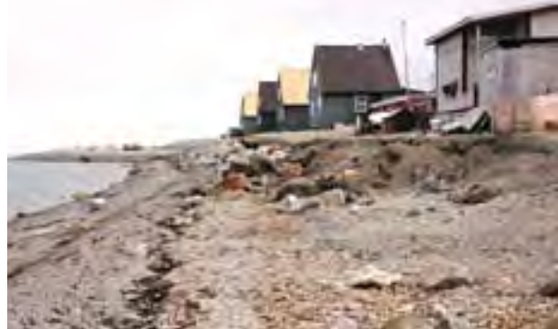
Figure 2. Erosion undermining houses and sheds along the waterfront at Hall Beach, NU, looking South. Erosion is occurring downdrift of a northward migrating gravel foreland in the background. Note collapsed seawall in middle distance. Local residents report significant reduction in sea ice and much later fall freeze-up, leaving more open water during the fall storm season. This may be contributing to increased erosion, despite a falling relative sea-level trend in Foxe Basin. Photo: D.L. Forbes, Geological Survey of Canada, 17 August 2007.
