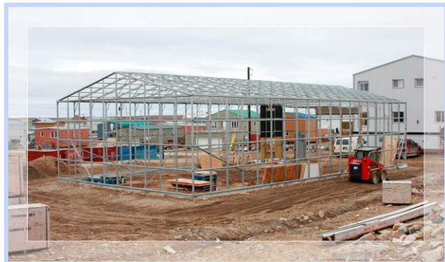
Steel frame construction in Cambridge Bay
