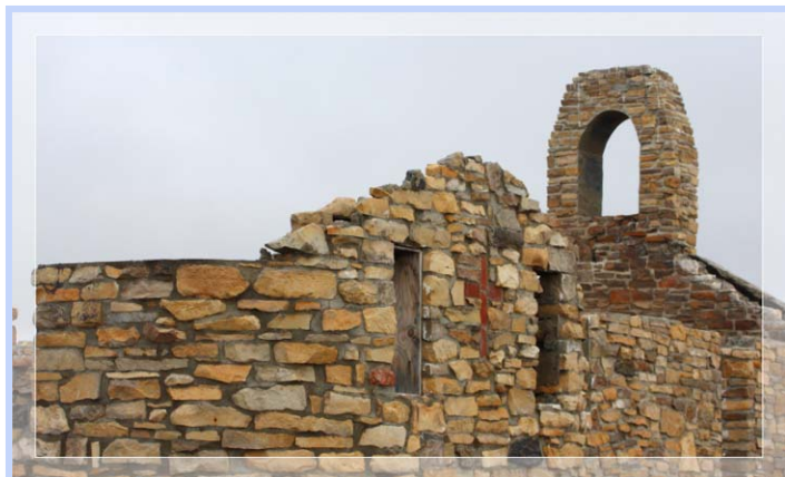
Church in Cambridge Bay built in 1953 using local materials of seal oil, clay and frost shattered rocks.
