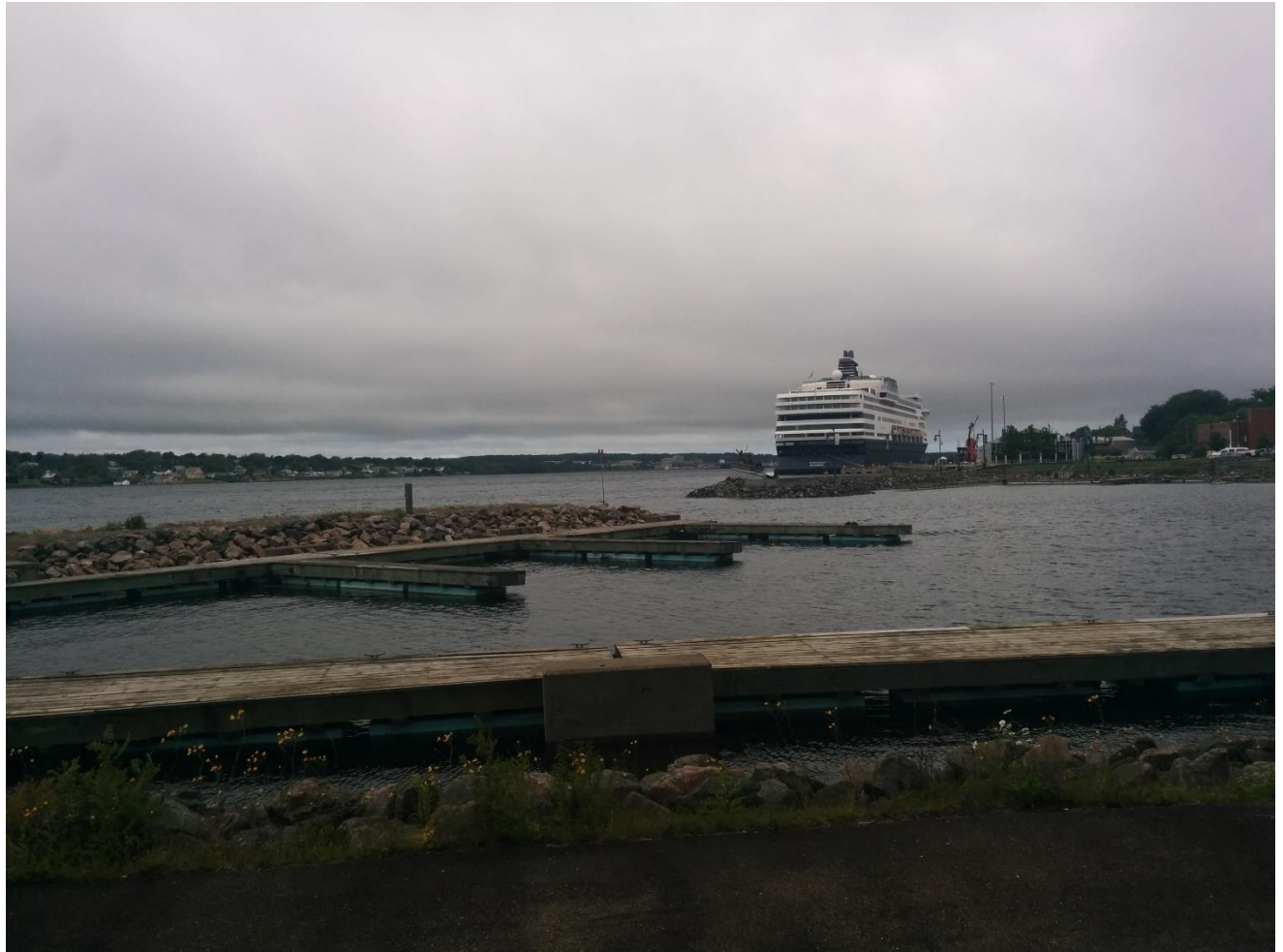
Figure 3-1: Marina Immediately to the South of the Sydney Marine Terminal
