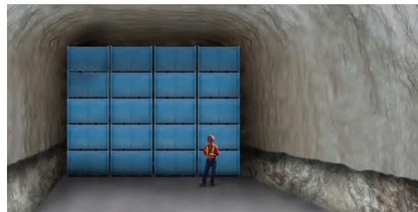
Low level waste emplacement room.
