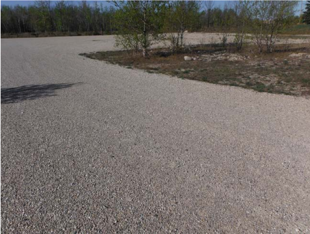
Plate 23: Recent gravel disturbance, facing south-west, May 7, 2013.
