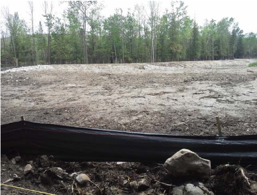
Plate 33: Construction area between complex and landfill, facing south, May 21, 2013.
