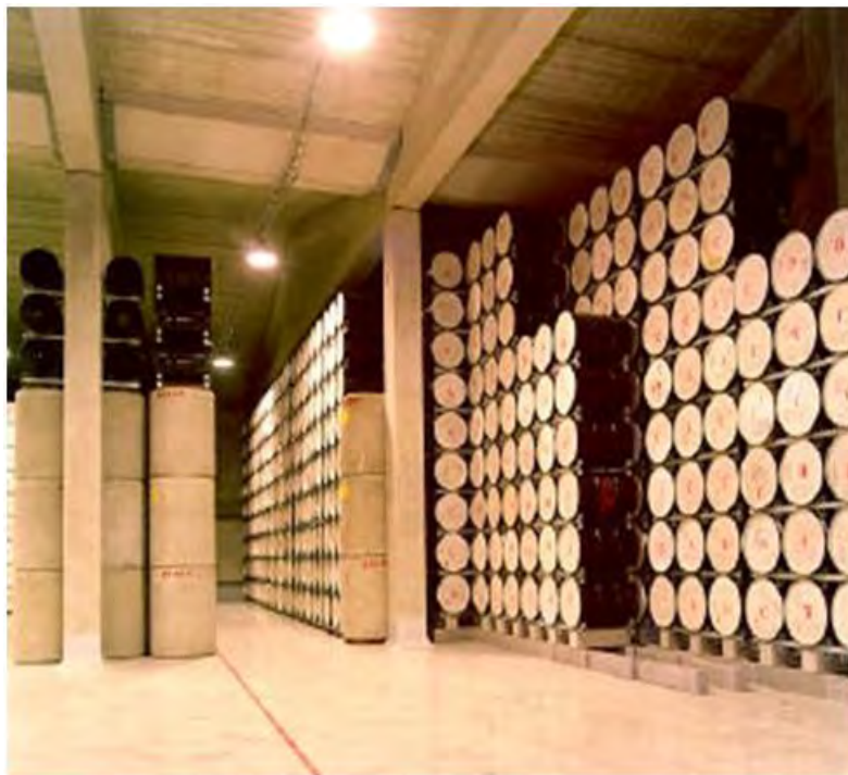
Figure 4.1: Photos of the long-term L&ILW storage building and containers at COVRA in Netherlands. Each building has a capacity for about 5000 m 3 of waste, has 40-cm thick concrete walls and a design life of 100 years.
