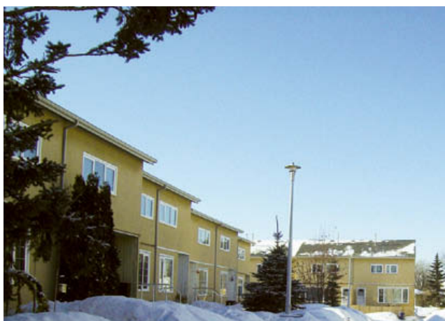
Synergen Housing Co-operative
