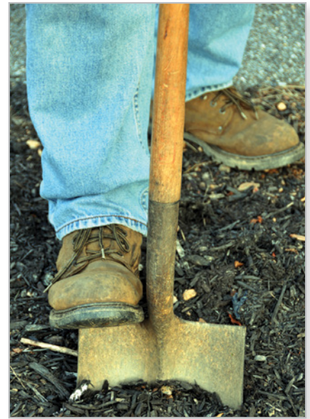
Figure 24 For your safety, make sure to contact local utilities before digging
