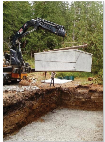
Figure 15 Concrete underground rainwater tank (10,600 L) being lowered into place
