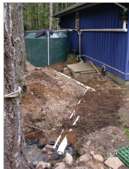
Figure 17 An overflow pipe discharges all excess water in an appropriate location away from foundations and other structures
