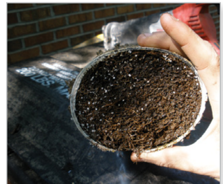
Figure 13 Failure to maintain eavestroughs and downspouts can lead to problems: this downspout is completely clogged by accumulated debris and had to be replaced
