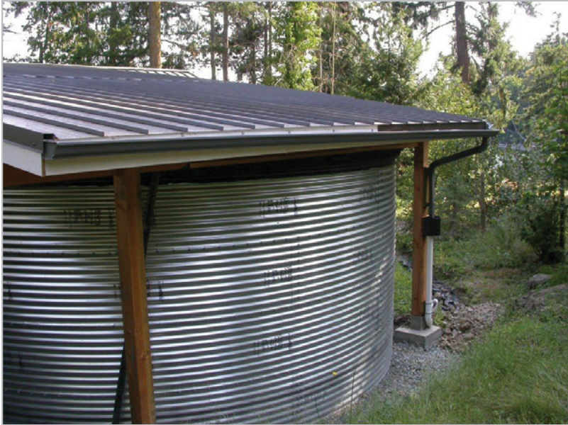
Figure 12 A properly sized and sloped eavestrough leads rainwater to the desired downspout, reducing the occurrence of water overflows
