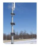
The new Sarnia truck inspection station has a combined windmill/ solar application. The 5KW system supplements MTO's power needs, and when not needed, the power is fed into the provincial grid.
