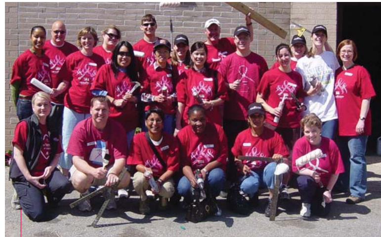
CIBC employees participated in a United Way Day of Caring at the Jane and Finch Boys and Girls Club in northwest Toronto. Volunteers helped in the renovation of "The Garage", an old garage that is being converted into 1,800 square feet of programming space for youth in this neighbourhood.
