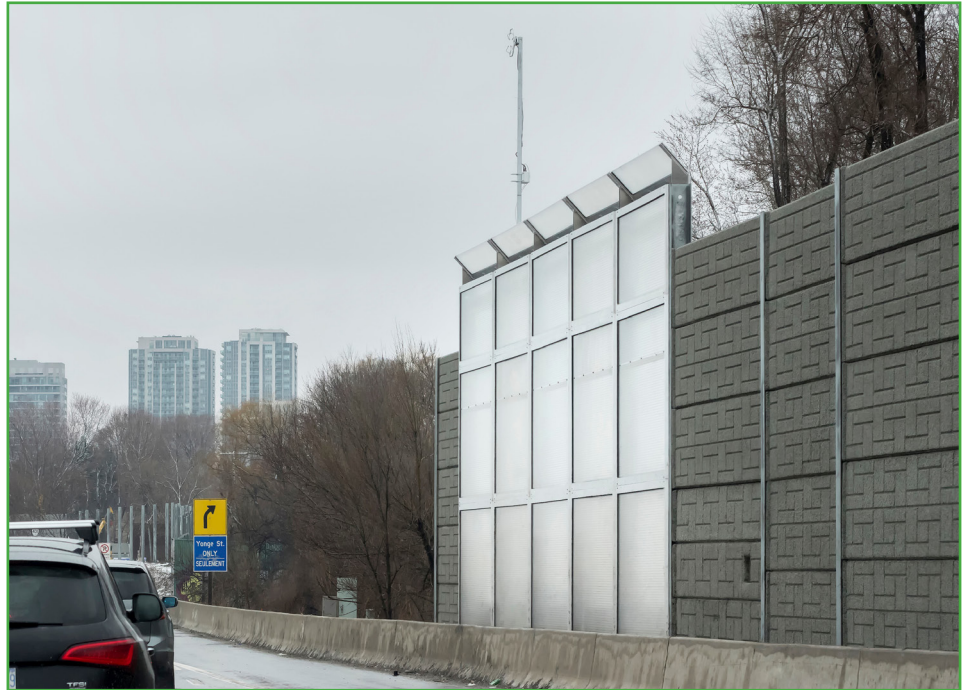
A 15-metre section of SmogStop™ acrylic noise barriers installed on the north side of Highway 401 during a rehabilitation project in 2017
