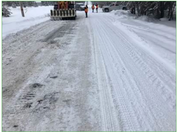
Figure 5: The results of snow and ice cleared from an Ontario provincial highway using Snow Lion equipment. Divots are visible in the remaining one centimetre of snow. These divots assist in retaining salt and sand on the road.
