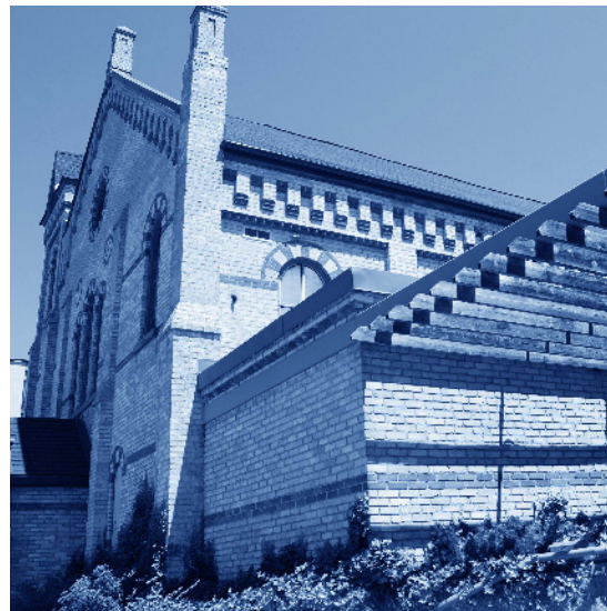
The former South Water Street Baptist Church in Cambridge was converted into a theatre in 1980. It continues to operate as the Cambridge Arts Theatre, a performance space for Galt Little Theatre. The successful adaptation illustrates the compatibility between original church design and subsequent use as a performance venue. (Photo courtesy of City of Cambridge)
