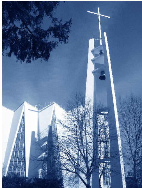
The Pines Chapel in Chatham-Kent is a stunning example of modern architecture. The triangular stained glass windows protrude from inverted white concrete walls and rise to form a crown. The Chapel was evaluated by the municipality and designated under the Ontario Heritage Act for its design and contextual significance. (Photo courtesy of Municipality of Chatham-Kent)
