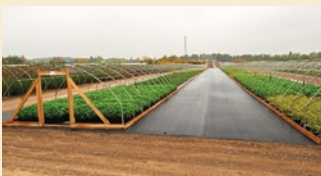
A well-designed container bed and runoff collection system – with suitable slopes and protected collection channels – will divert irrigation runoff for collection.
