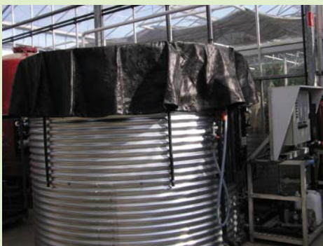
Ozonation uses ozone, an oxidant with twice the effect of chlorine, to destroy pathogens and other microbes.
