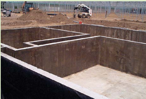
This below-ground reservoir can store fresh water, nutrient feedwater, or disinfected or treated leached nutrient feedwater.
