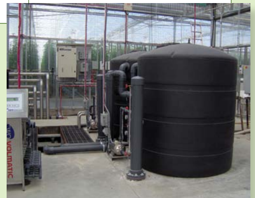
Ozonation uses ozone, an oxidant with twice the effect of chlorine, to destroy pathogens and other microbes.
