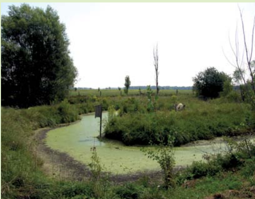
Constructed wetlands will reduce particle and nutrient levels of post-production wastewaters.
