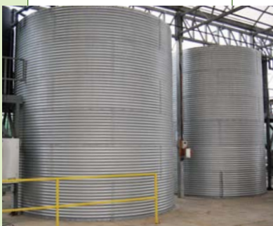
Leached nutrient feedwater is nutrient-rich and should be collected and stored separately from other greenhouse wastewaters.
