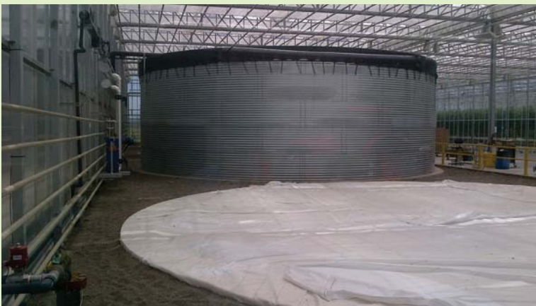
Store irrigation water in leak-proof containers such as above-ground, lined storage tanks.
