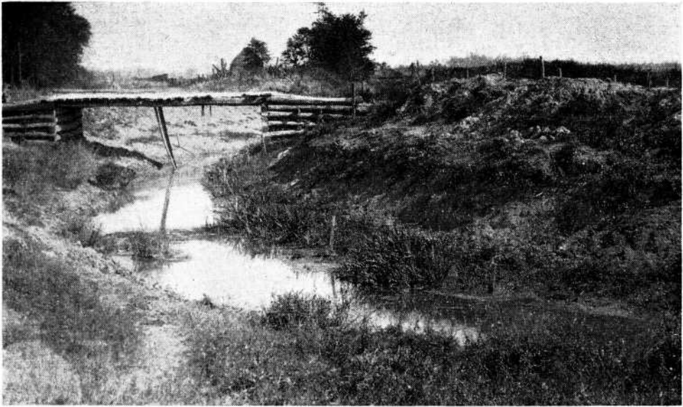
Large open ditches provide outlets for tile on broad areas of nearly level land.
