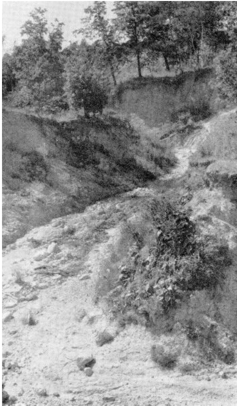
Gully-erosion is often a problem along the lakeshore.
