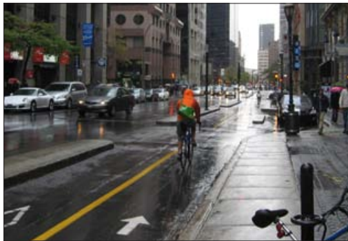
Physically-separated curb-side bike lanes such as this example from Montreal create a safe and secure dedicated environment for cyclists along busy streets.
