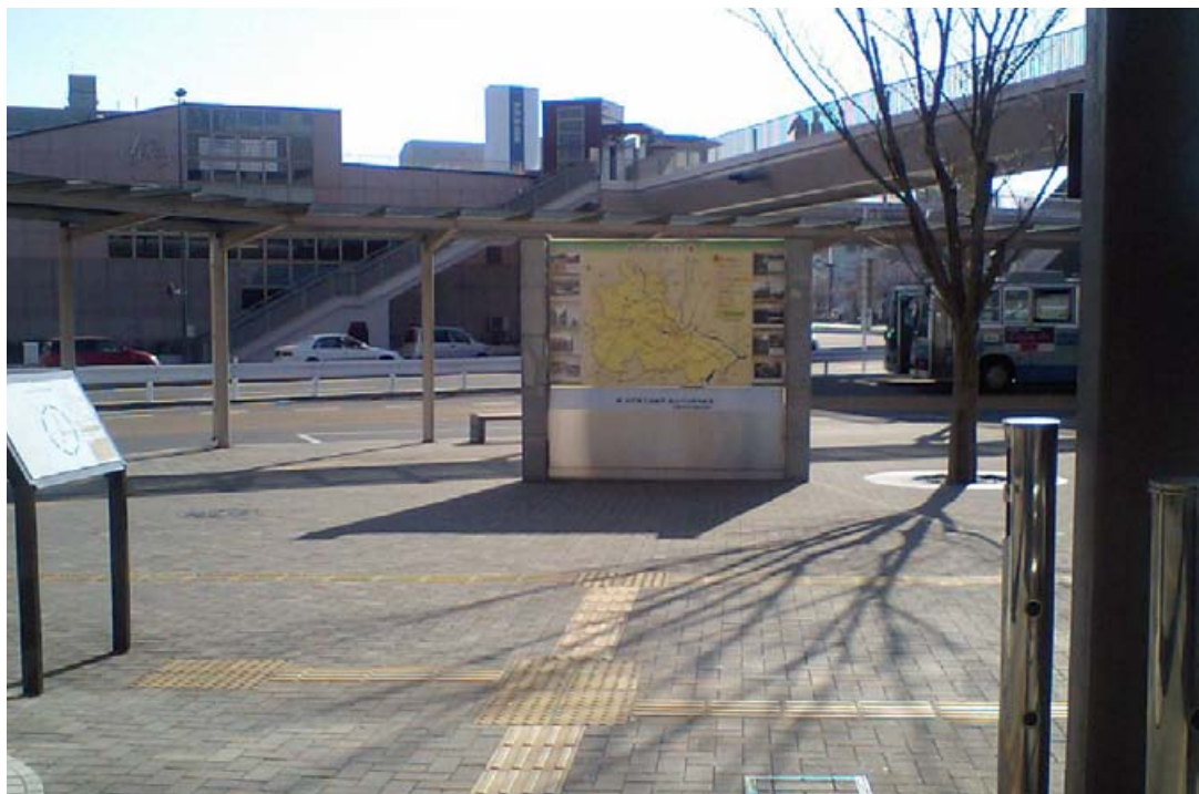
The paving and signage at a bus station in Tokyo are used together to direct both seeing and visually impaired passengers between the various parts of the station.
