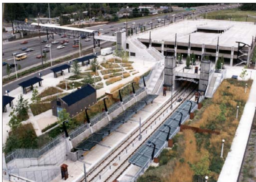
The Sunset Transit Center in Oregon is a major transit hub bringing together, LRT, bus, park and ride and cycling facilities. The Center has been designed to create a welcoming environment for users with high-quality architecture and the integration of a signature open space.
