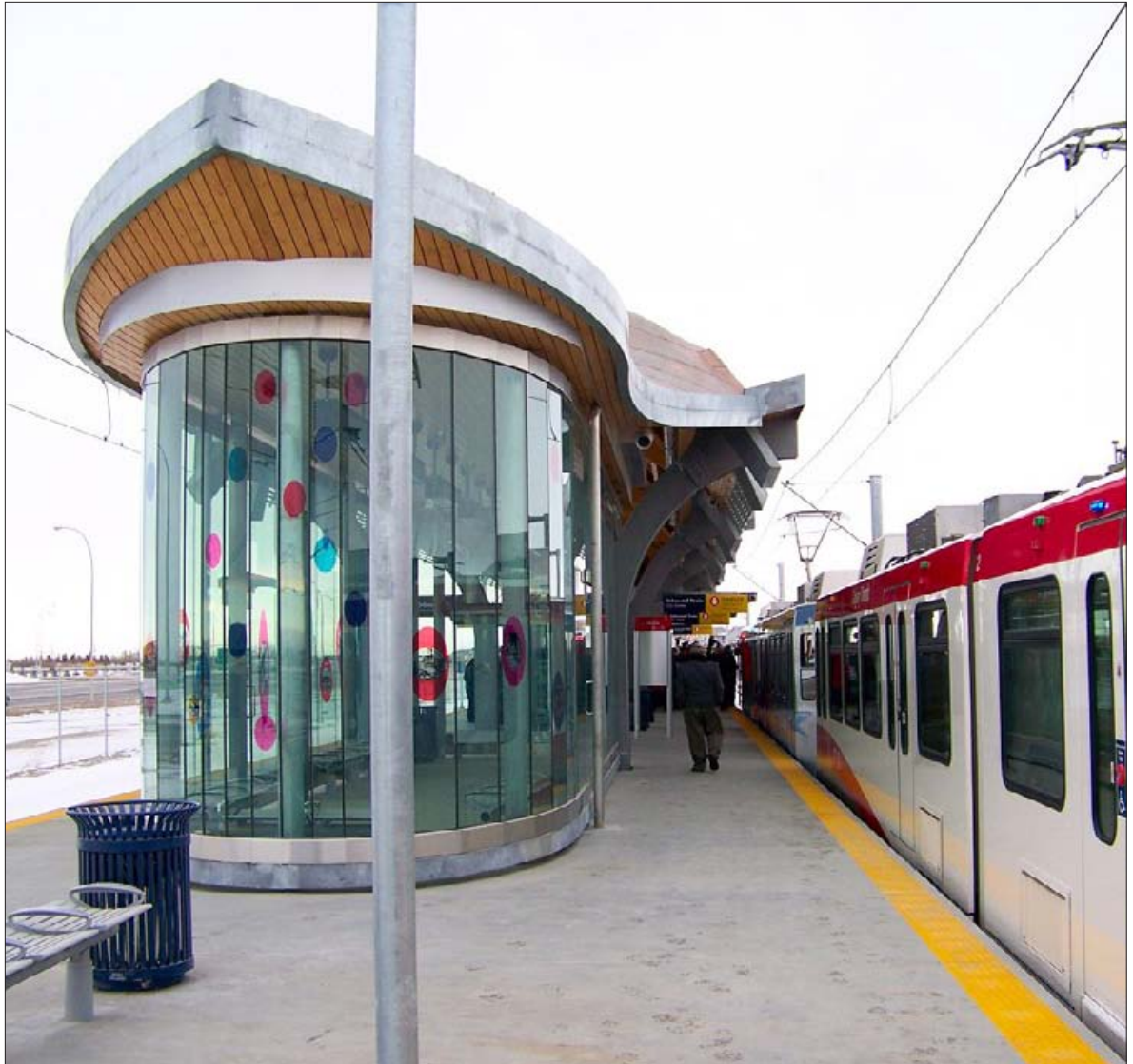
The use of glass in this shelter in Calgary, Alberta enhances natural surveillance and lighting.
