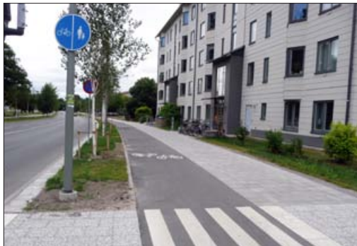
Dedicated bike lanes adjacent to sidewalks such as this Stockholm example create a safer environment for cyclists and facilitate plowing during winter months.
