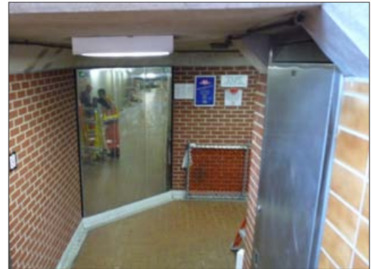
When blind corners are unavoidable, a mirror like the one used at this GO Station allows visibility around corners.
