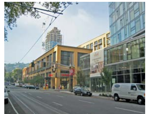
Light rail expansion in Portland, OR, has spurred the development of new residential neighbourhoods along the length of the route.
