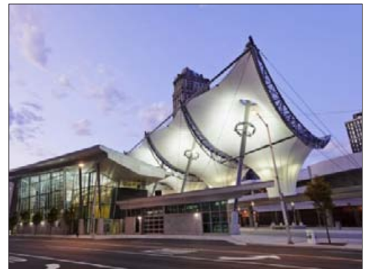
Detroit’s Rosa Parks Transit Center not only integrates several modes of transit, it creates a local landmark that helps to raise the profile of the city’s transit service.
