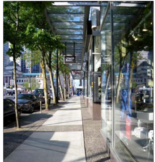
Street-related buildings can contribute to pedestrian comfort through the provision of canopies that can mitigate against the impacts of wind or weather.
