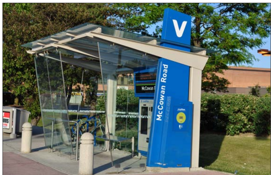
This transit stop in York Region is composed of high quality materials that provide clear sightlines to surrounding areas. The shelter provides real-time trip planning information and incorporates a ticket vending machine for pre-paid boarding. Users are supported through amenities such as seating, waste receptacles and bike racks.
