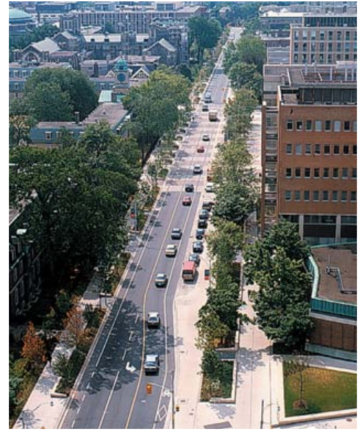
St. George Street running through the heart of the University of Toronto campus was rebalanced in 1997 through the addition of bike lanes and pedestrian-supportive paving treatments to create a street that better supports the many pedestrians and cyclists that use it daily.
