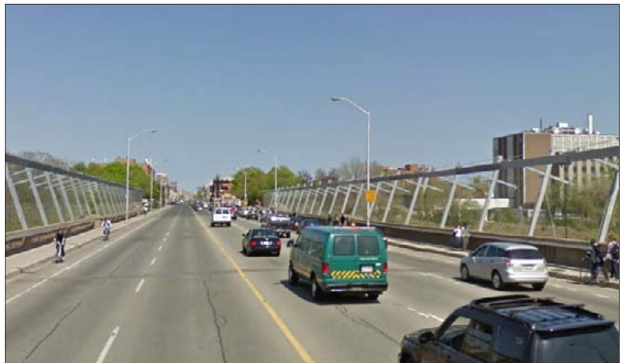
Though a major thoroughfare, the Prince Edward (Bloor) Viaduct in Toronto has been designed to accommodate motor vehicles, pedestrians and cyclists, and includes a separate level beneath the road to accommodate subway trains.
