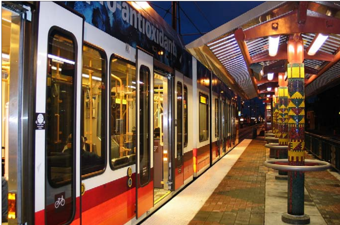
North Killingsworth LRT station in Portland, OR, provides a variety of seating and standing options with incorporated public art for passenger enjoyment.
