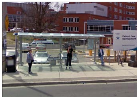
The new bus shelters along the iXpress routes contain EasyGO displays to provide real-time departure times for buses. Bike racks are provided adjacent to the shelters to encourage people to ride to the stops, which are spaced further apart than for non-express routes.
