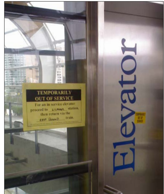
Poor maintenance and life cycle management can lead to system failures that create inconveniences for passengers.
