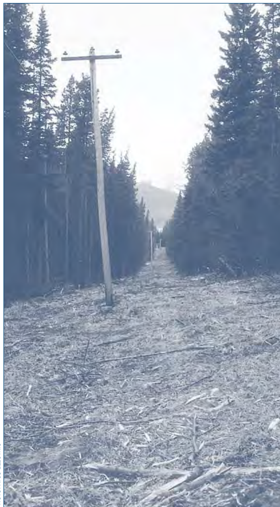
PHOTO: ATCO ELECTRIC
