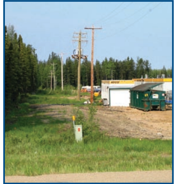
Illustration of hazard tree removal on powerline.
